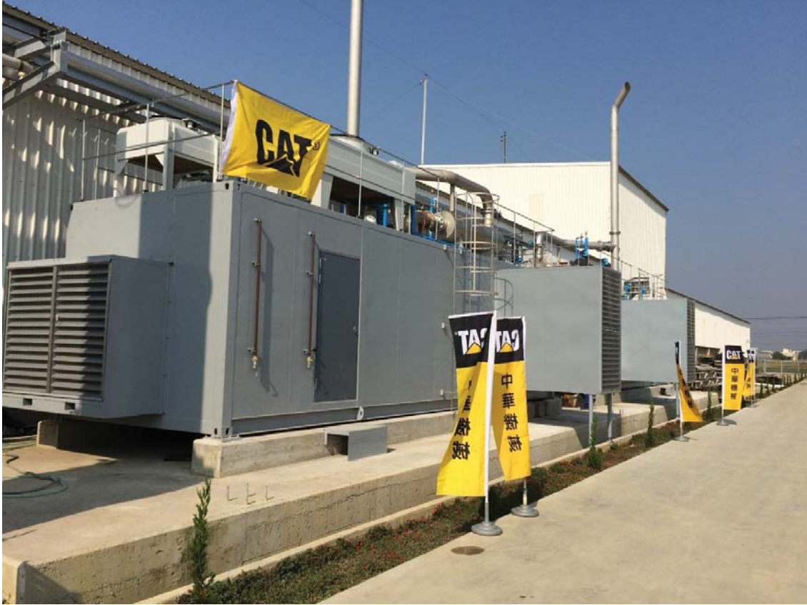
Figure 17: ShiAn Tainan Project: Cat CG132-08, 2x 400 kW biogas generator sets in 54 dBA (10 m) sound enclosure.
