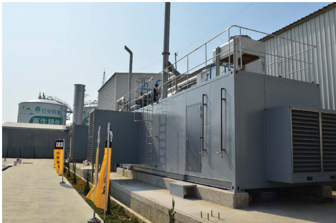
Figure 16: ShiAn Tainan Project: Cat CG132-08, 2x 400 kW biogas generator sets in 54 dBA (10 m) sound enclosure.
