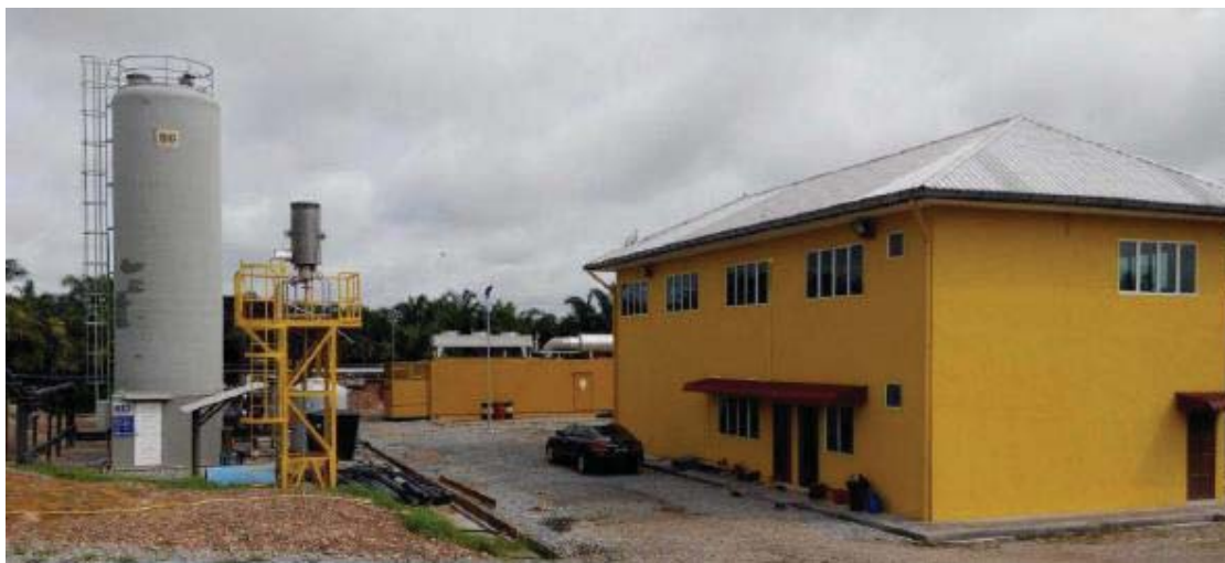
Figure 26: Jeng Huat Kemayan project: Site overview.
