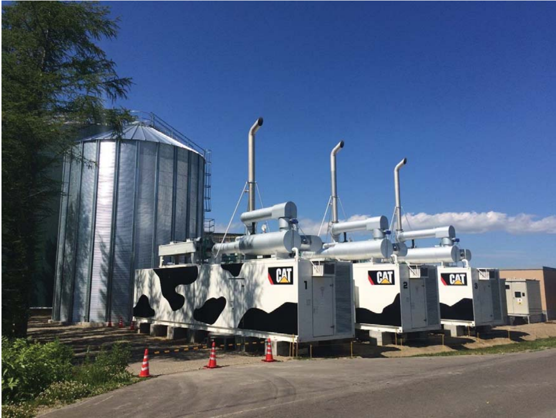
Figure 6: MES Hokkaido biogas-to-power project: Cat CG132-12, 3x 600 ekW biogas generator sets in containerized sound enclosure (85 dBA at 1 m).
