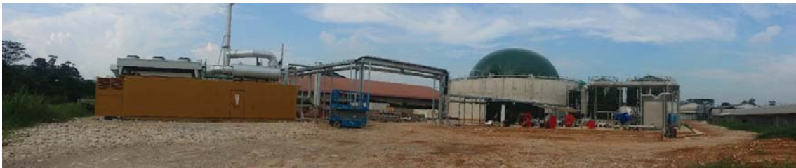
Figure 21: Anaergia SCCF Singapore project: Site overview.
