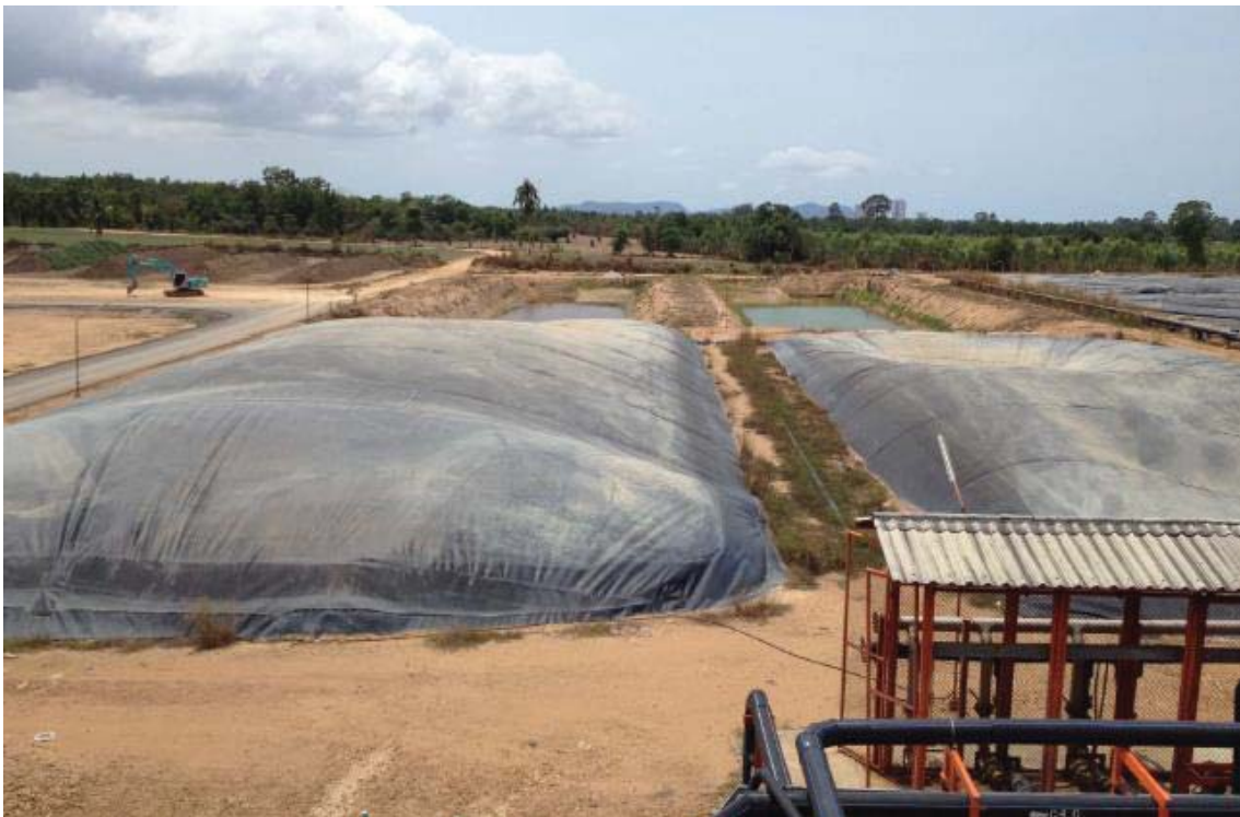
Figure 27: TQS Kanchanaburi project: Lagoon digesters.
