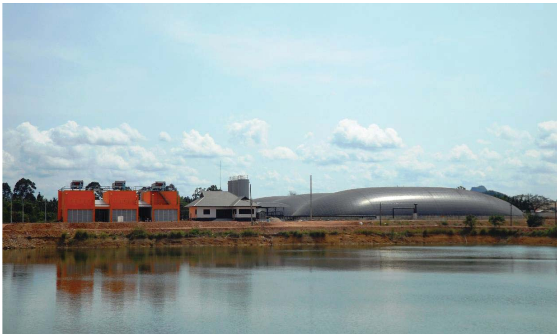
Figure 31: HEMCO PPG site overview.
